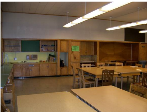
Main building (274A), classroom, looking south.
