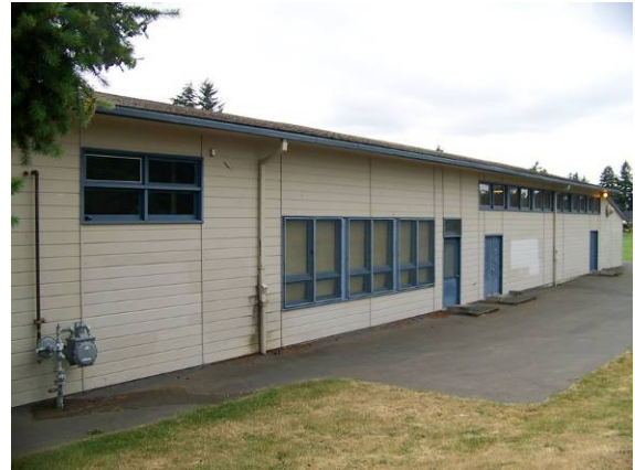
Main building (274A), north (rear) elevation, looking southwest.
