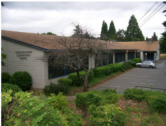
Main building (274A), south (front) and east (side) elevations, looking northwest.
