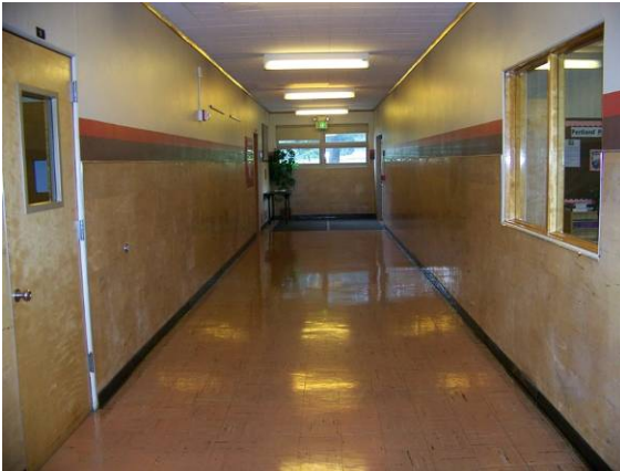
Main building (274A), rear hallway at office, looking east.
